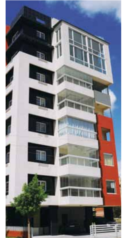
Salim Khalil Building Location: Badaro
